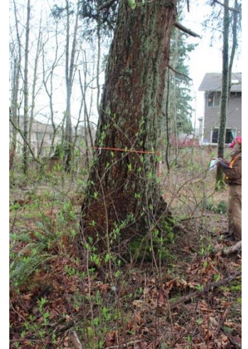
Sloughing bark, horizontal crack with lean
